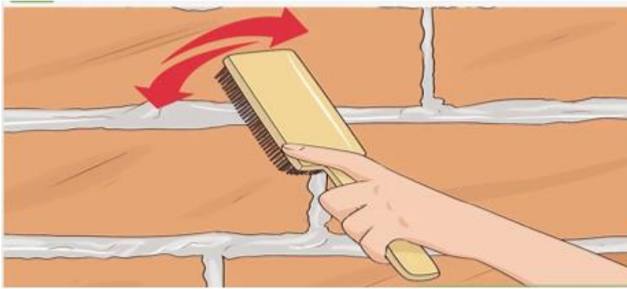
Fig 6. Wipe off excess mortar
