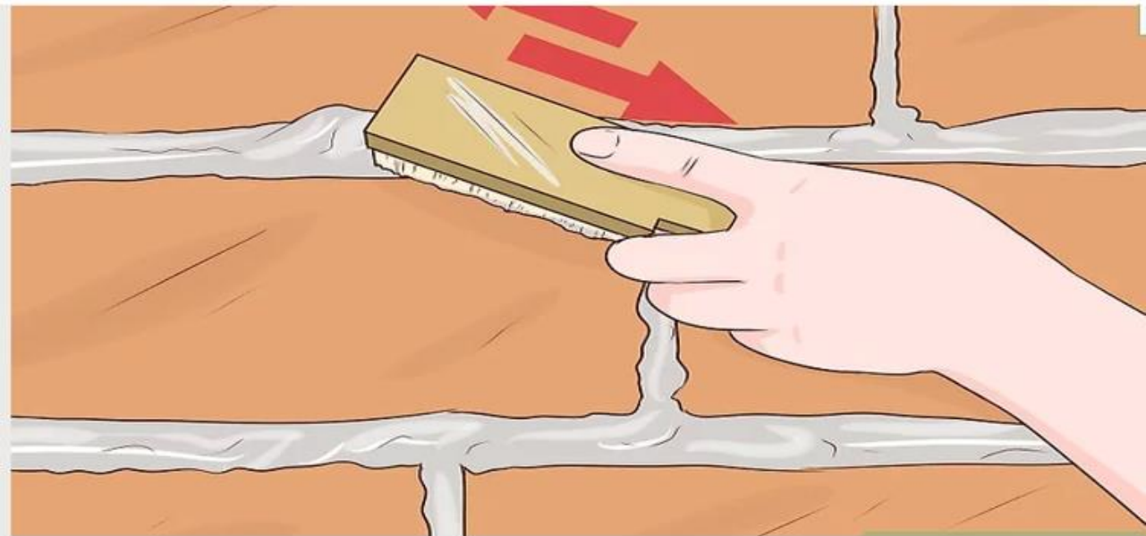
Fig 2. Rub off remaining mortar
